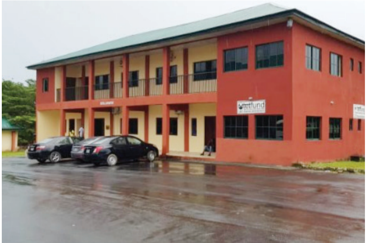
Completed TETFund building at UNICAL
